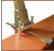
Stanchion installation complete
